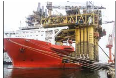
Synchronous superlift and launch
