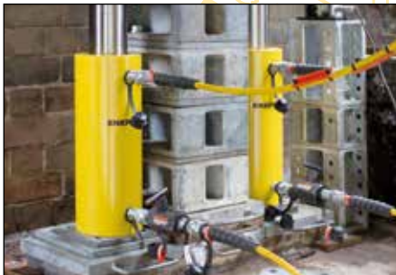
Bridge lifting and launching
