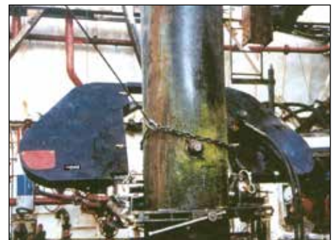
▼ Decommissioning job with band saw.
