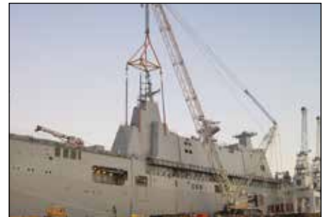
Synchronous hoisting and load positioning
