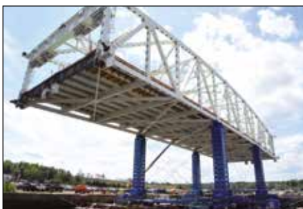
Incremental bridge lifting
