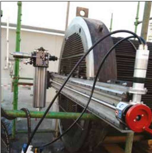
▼ MRY Milling machine on a heat exchanger.
