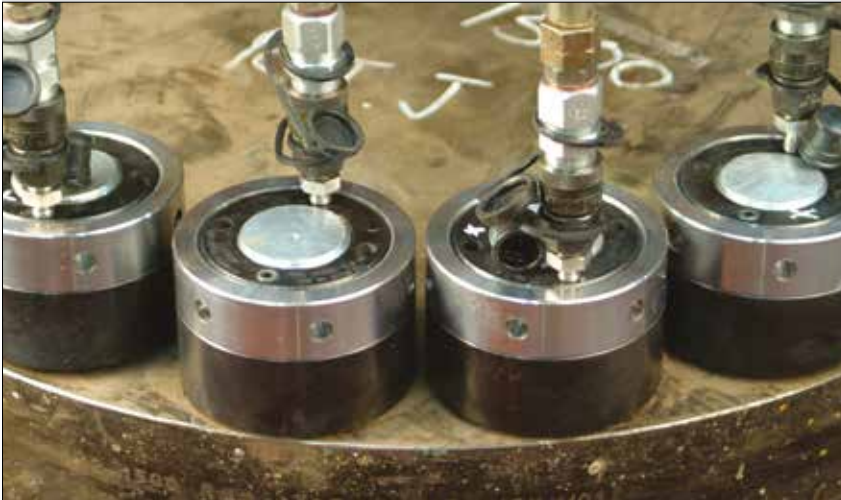
▲ Tensioning with hydraulic nuts.
